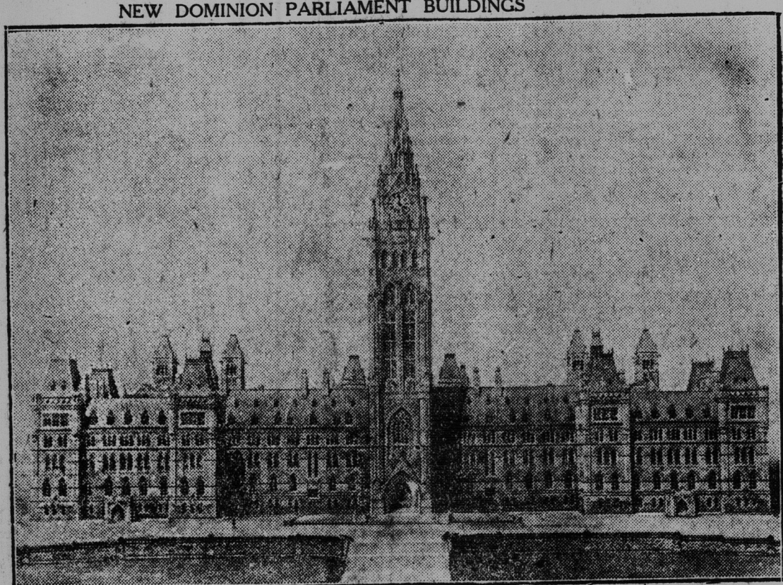
A splendid view of the new House of Commons structure at Ottawa in course of construction.
