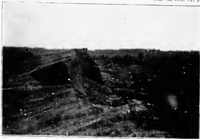
FIGURE 1.—NORTH EDGE OF LANDSLIP AREA, VIEWED EASTWARD FROM NEAR THE OUTLET
