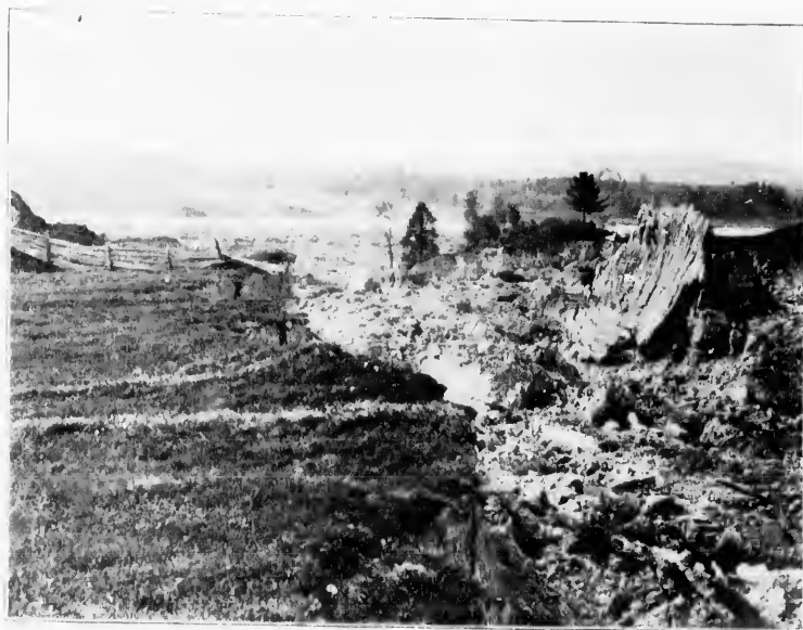
FIGURE 2.—OUTLET OF LANDSLIP, LOOKING TOWARD BLANCHE VALLEY
