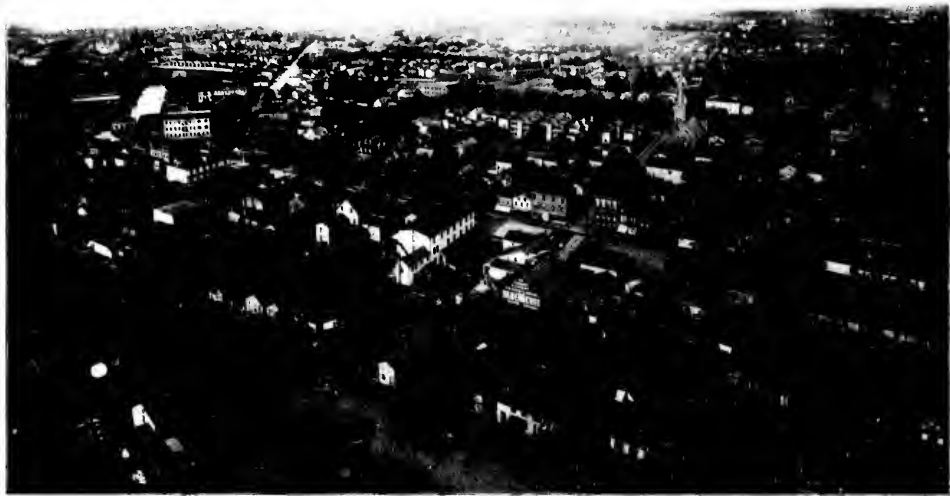
FROM THE OVERLOOK TOWER — LOOKING EAST
