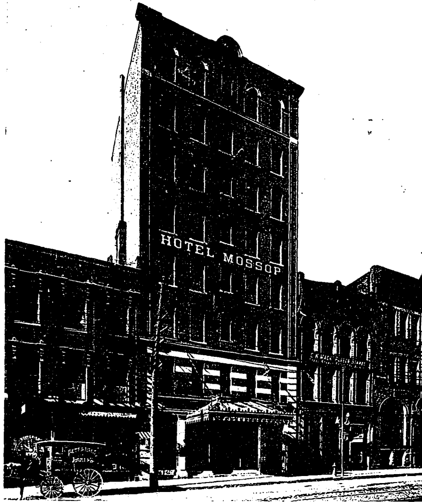
Hotel Mossop, Toronto, which, both externally and internally, is of absolute fireproof construction. It stands on a foundation of 18 concrete wells, carried down to bed-rock, the first foundation of its kind to be installed in Toronto. J. P. Hynes, Architect.
