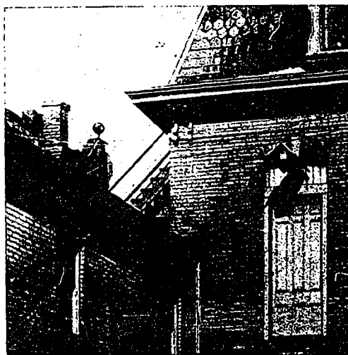
The only fire escape on a Toronto school building; a wooden affair that runs down from the third story of the York Street School to the roof of another building. This was erected about the time of the Collinwood disaster.
