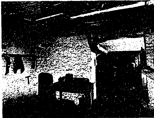
One of the "fireproof" basements in Toronto schools. It will be noted that it has not even metallic ceilings, and the furnace pipe runs directly under a wood beam above the doorway. The only protection being afforded is a piece of tin between the pipe and the beam. There is a can of oil under the table, which would contribute toward the "fireproofing" of this room.
