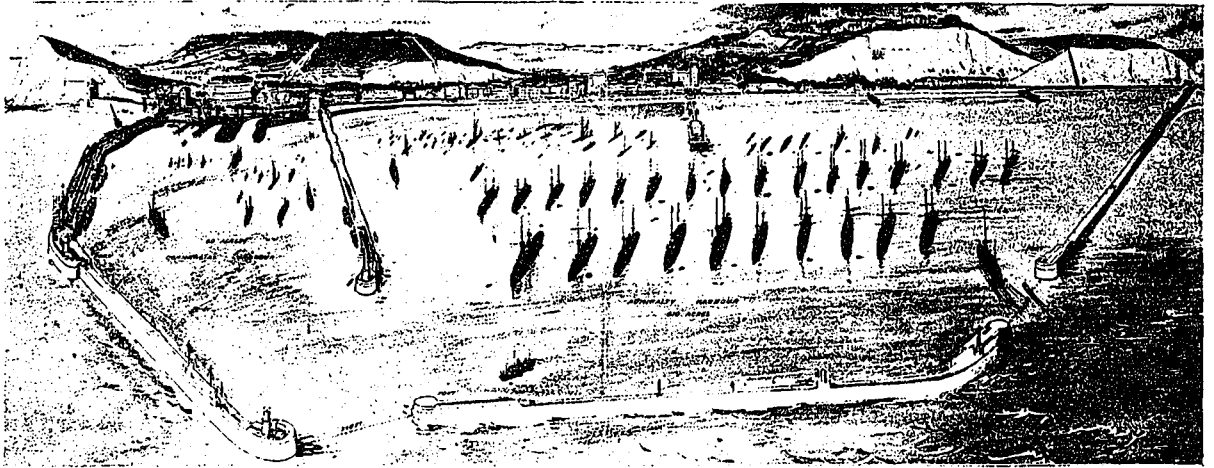
The new Harbor at Dover, as seen from the English Channel, the greatest artificial enclosure for war vessels and merchantmen ever constructed. Some idea of the magnitude of the undertaking may be gathered from the fact that the outer masonry walls alone measure 2\frac{1}{2} miles in length, and necessitated in their construction over a quarter of a million barrels of Portland cement.
