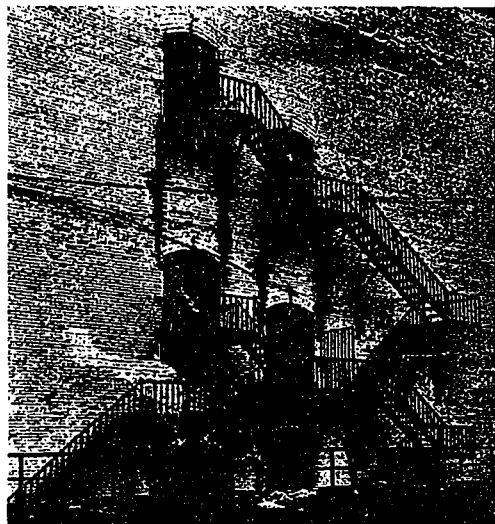
The system of outside stairways with which the Royal Alexandra Theatre is equipped. If theatre-goers are entitled to this fire protection, we ask why our school children should not receive some consideration.
