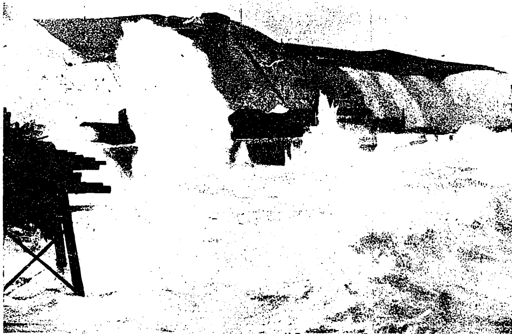
One of the many difficulties contended with in building Dover Naval Harbor. The point at which the work was carried out is one of the roughest spots of water between England and France, being exposed to all seas from east to west. In order to place the massive concrete blocks, it was necessary to erect for temporary use a ponderous wooden staging, on huge piles of a special wood brought a distance of 13,000 miles.
