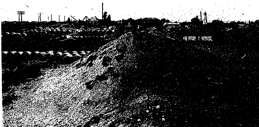
View showing sections of the huge concrete pipes which will form the conduits through which the raw and filtered water will flow. The manner of laying and locking the joints of these pipes will be one of the most interesting processes of the work.
