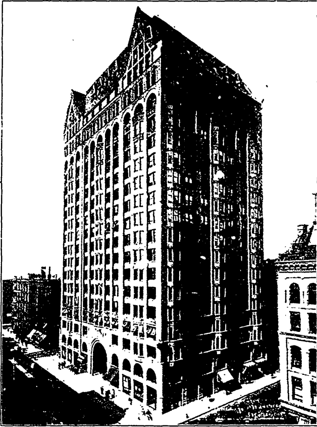
STEEL STRUCTURE—MASONIC TEMPLE, CHICAGO.
