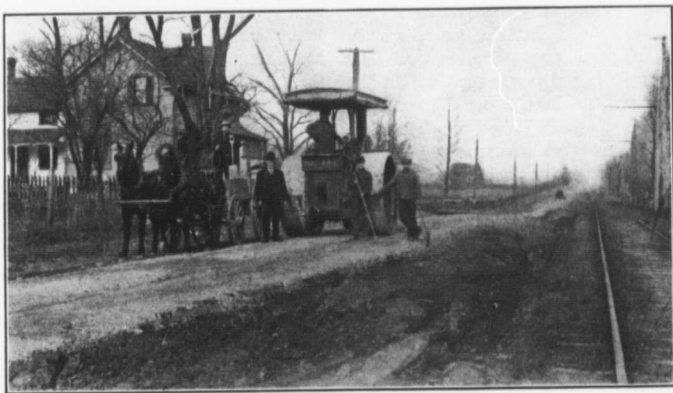
INTELLIGENT ROADMAKING. Peel County steam roller, near Port Credit.
