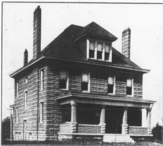
A COSY COUNTRY HOME. The blocks are made on a London Face Down.
