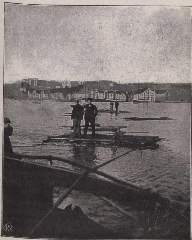
Fig. 4.—Sinking Gas Mains.
