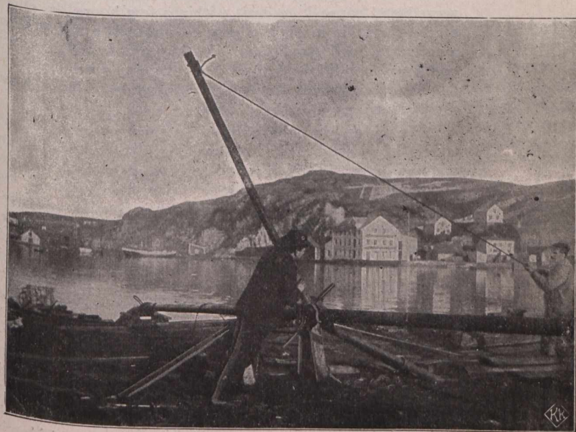
Fig. 5.—Screwing up the Joints of the Pipes.
