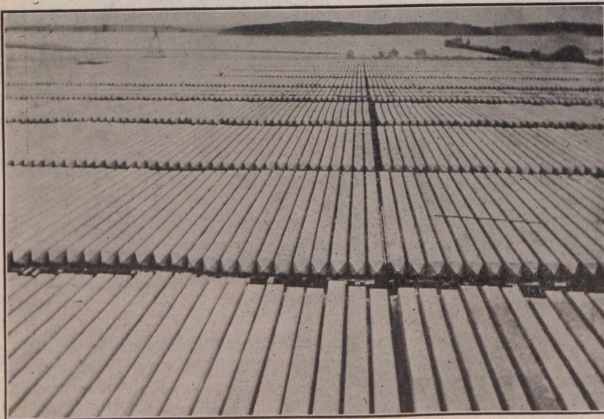
Fig. 4.—View of Pile Casting Yard.
