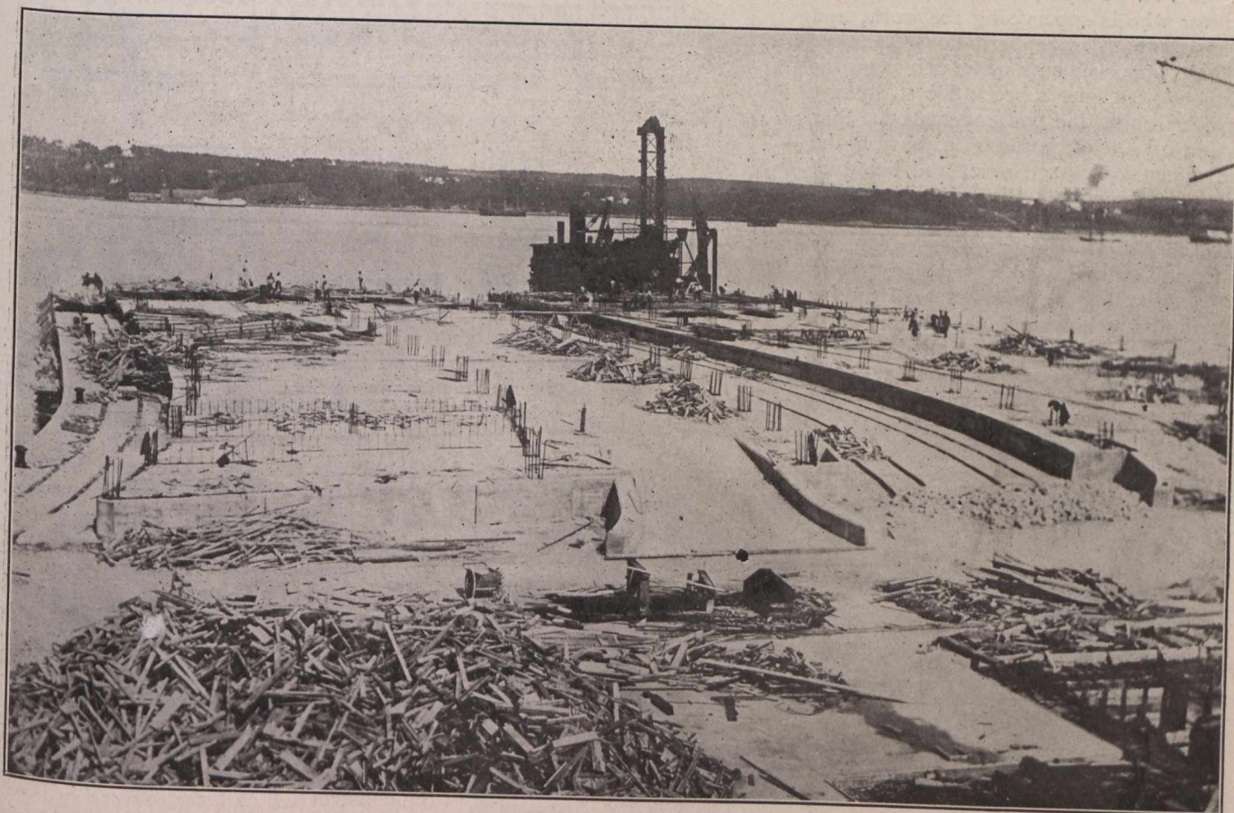
Fig. 1.—View of Pier No. 2 While Under Construction
