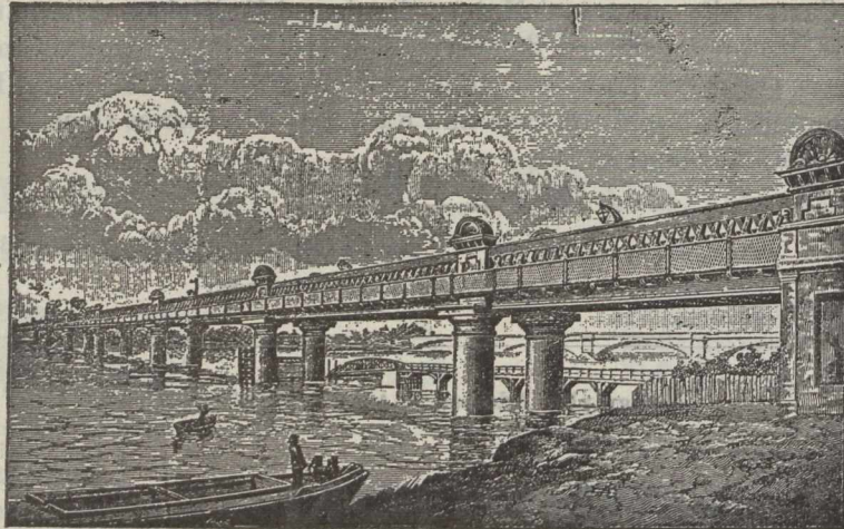
PUTNEY BRIDGE, OVER THE RIVER THAMES, LONDON.
