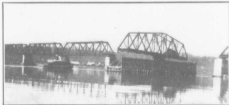
Railway Bridge on Fraser at Industrial Mission.
