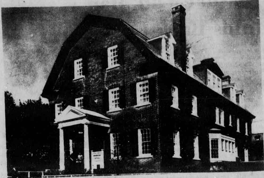
Beaverbrook House is the Saint John equivalent of Sir Howard Douglas Hall. It forms the core of the Saint
