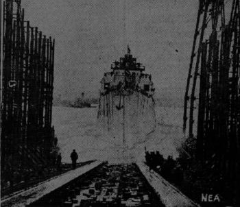
The Memphis (above) scout cruiser, launched in Philadelphia, is one of 10 ships of this class either launched or in process of building for the United States. She is 550 feet in length, has a speed of 40 miles an hour and is fitted to carry and launch airplanes.
