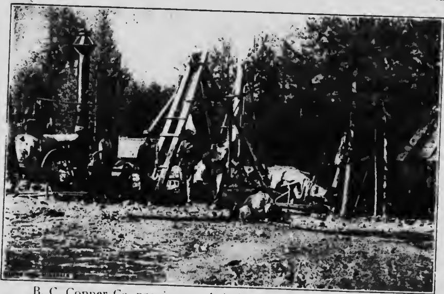
B. C. Copper Co. proving up their bonds on Copper Mountain by Diamond Drills.
