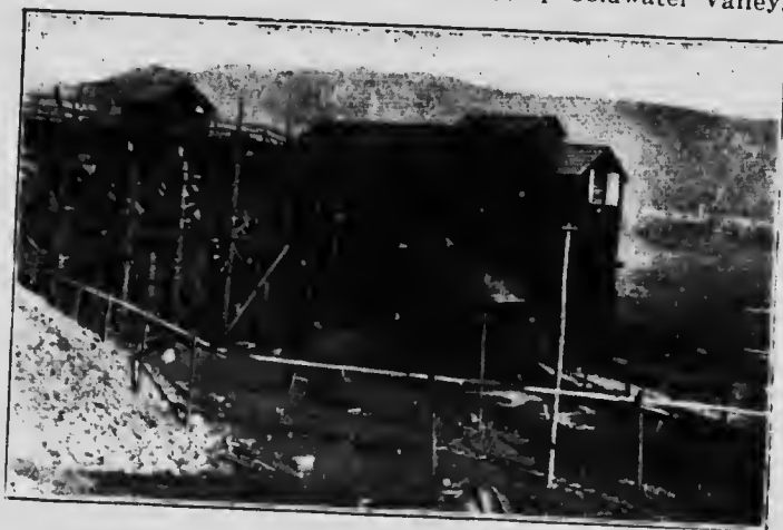
Fig. 4.—Near View of No. 1 Tipple.
