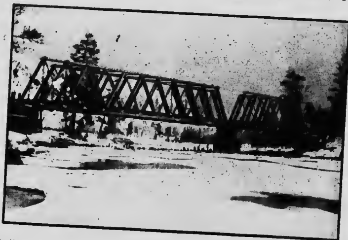
Railway Bridge across the Similkameen River near Princeton.
