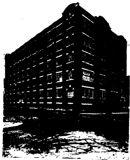
Southam Press Building, Toronto. Messrs. Sproatt & Rolph, Architects. W. J. McGuire, Ltd., Plumbers.
