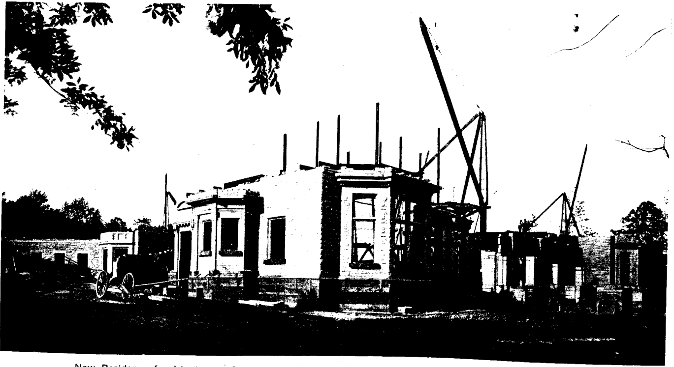
New Residence for Lieutenant-Governor of Ontario, Toronto. Provincial Architect Heakes, Architect. Don Valley Brick and Porous Terra Cotta used.
