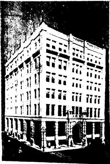
La Patrie Building, Montreal. Messrs. G. A. Monette and J. O. Turgeon, Architects. D. Ouimet, Plumber.
