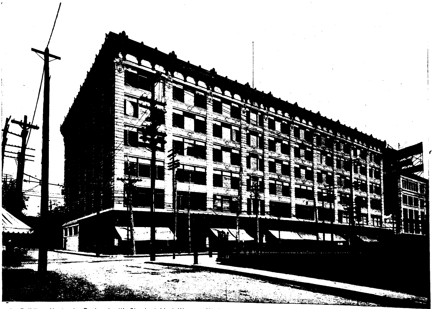
Jacobs Building, Montreal. Equipped with Standard Ideal Ware. Mitchell & Creighton, Architects. W. J. McGuire, Ltd., Plumbers.
