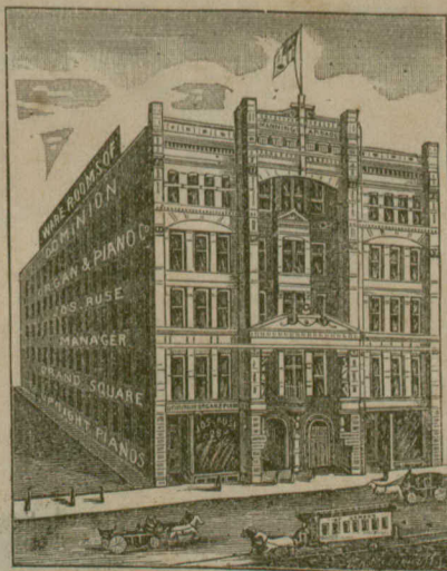
Our Warerooms in course of erection.
