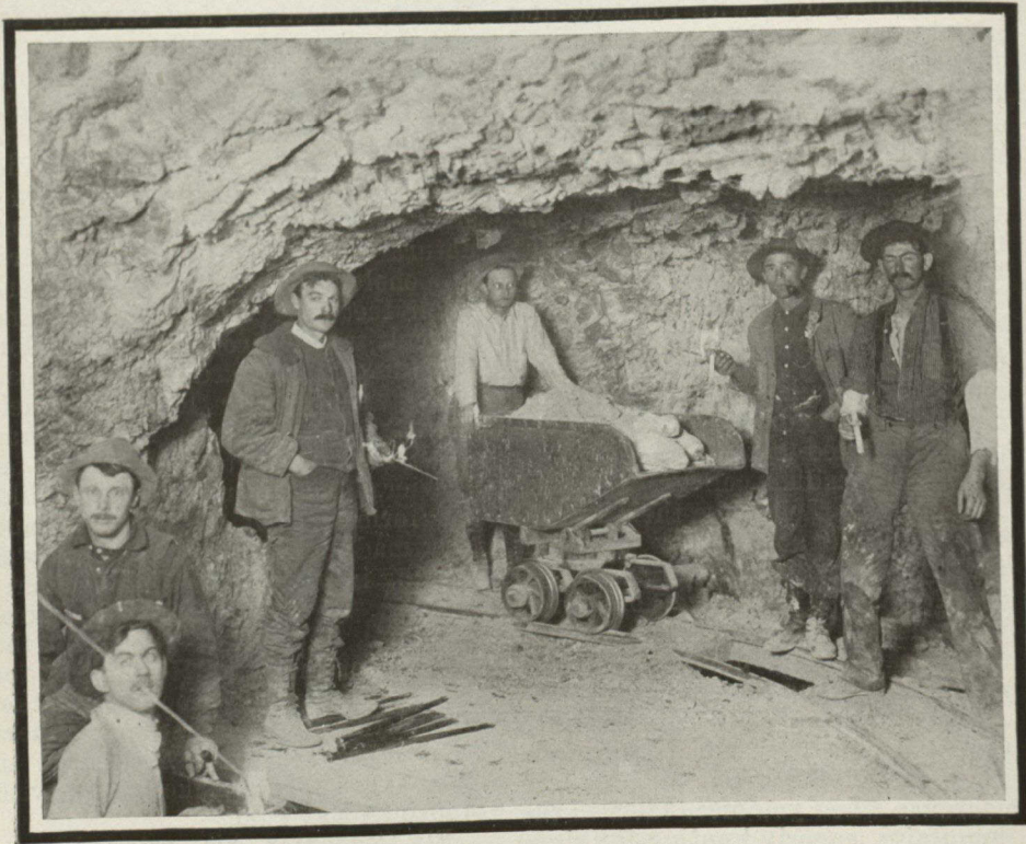
A TUNNEL IN A BRITISH COLUMBIA MINE
