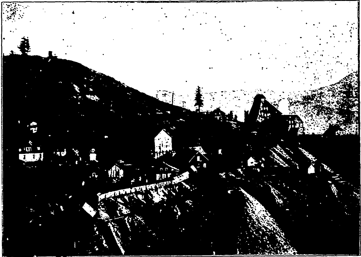
Rossland.—Le Roi Mining Co.'s Headworks over Main Shaft, in background.—Le Roi No. 2 Co.'s Josie Mine Surface Works and Dumps.
