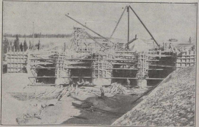
Headworks Under Construction, Showing Also the Riprapping of Canal Bank Before Surfacing With Concrete.
