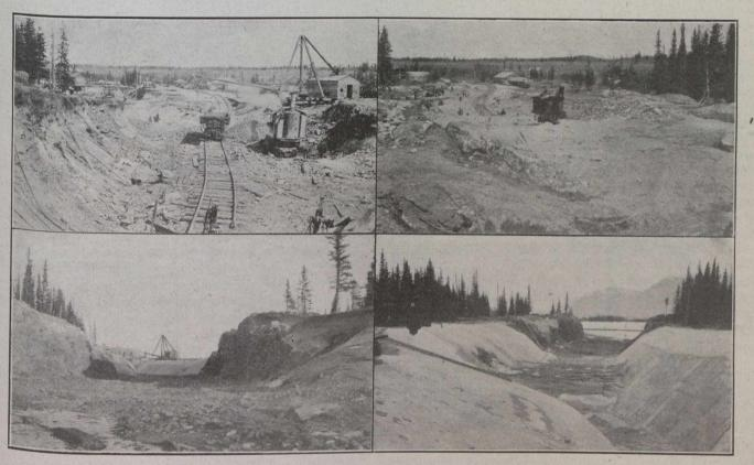
Views of Canal Construction at Kananaskis Falls. Excavation Looking Towards Headworks. Headworks Site from Canal Entrance. Steam Shovel Excavating Rock. Completed Canal from Headwork
