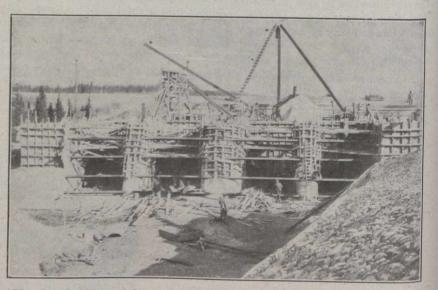
Headworks Under Construction, Showing Also the Riprapping of Canal Bank Before Surfacing With Concrete.
