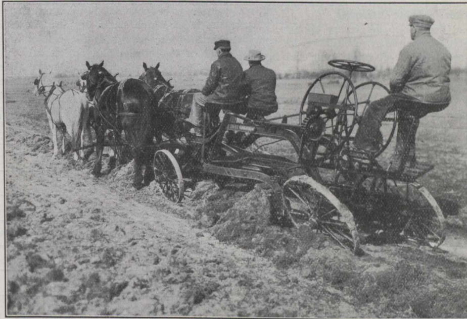
Grader throwing up first plowing.
