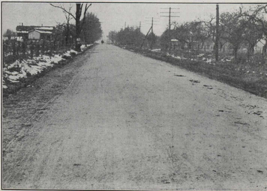
New York State Road between Rochester and Buffalo, paved with "Rocmac."
