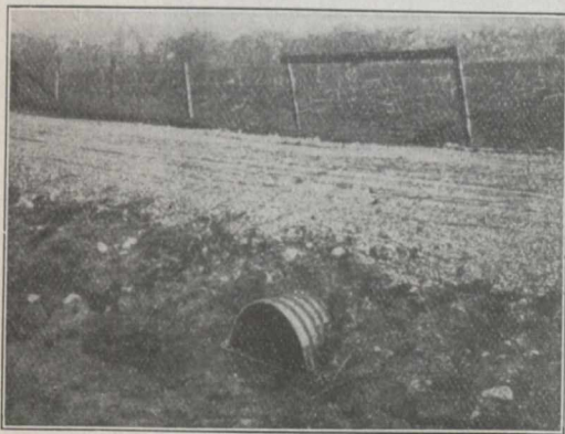
A 24-inch Corrugated Flat-Bottomed Culvert on a Highway, Where Conditions Prevented the Use of a Round Culvert of Proper Diameter for Required Drainage.
