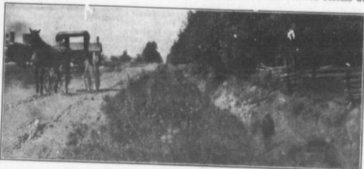
Large Sized Tile should be used in place of Deep Roadside Ditches.
