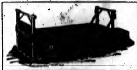
Outside View of the Andrews Progressive Kiln, showing Lumber placed crosswise the building, on Cars.
