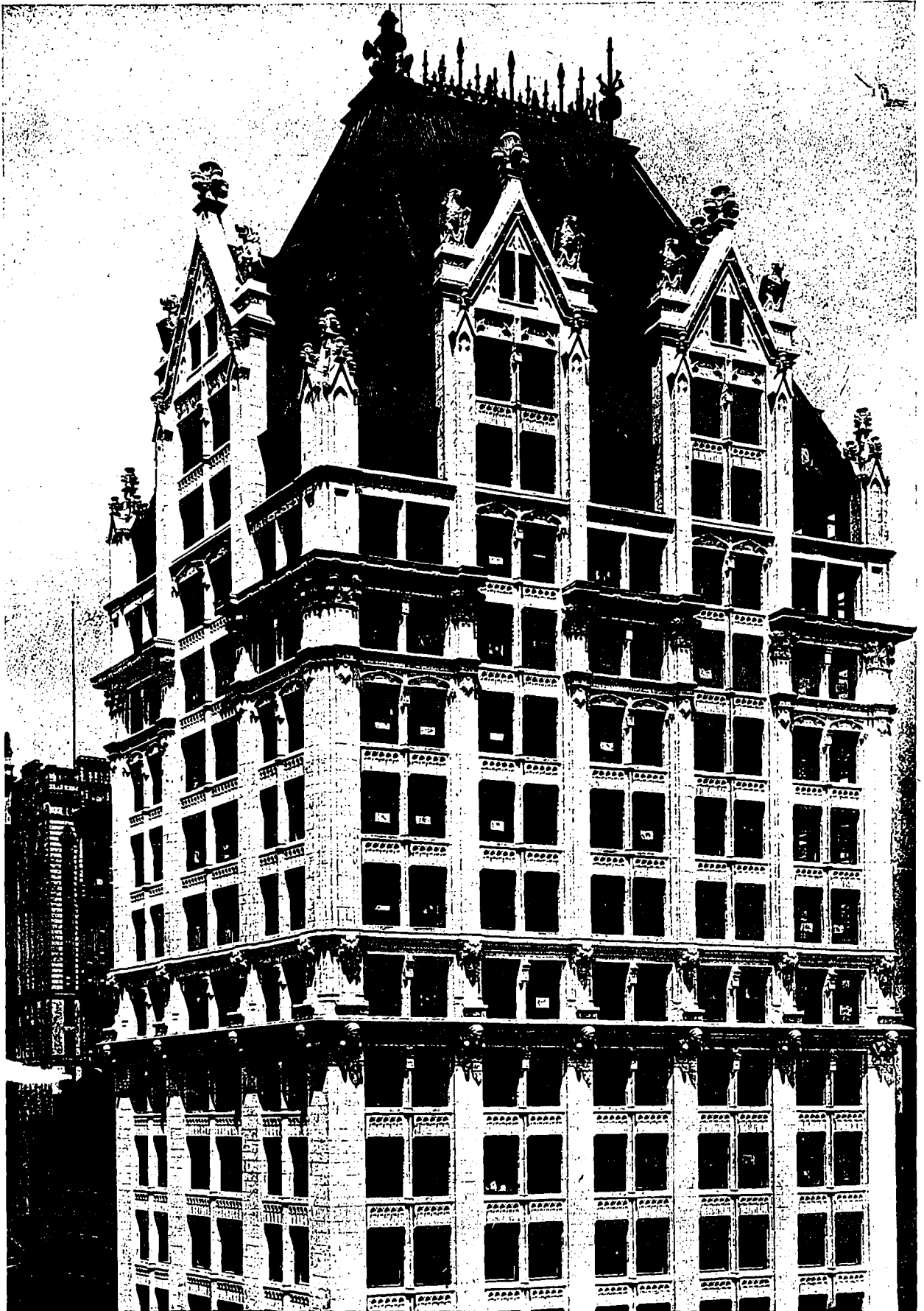
Liberty Tower, New York.—View of Upper Stories, Showing the Detail of Cornice and Pinnacles, together with the Treatment of Roof and Apex. Henry Ives Cobb, Architect.
