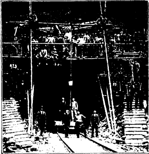
Ruppertsberg Tunnel, 1 mile long, constructed by the German Government, waterproofed with Ceresit. (This is only one of the many tunnels which have been waterproofed with our material.)
