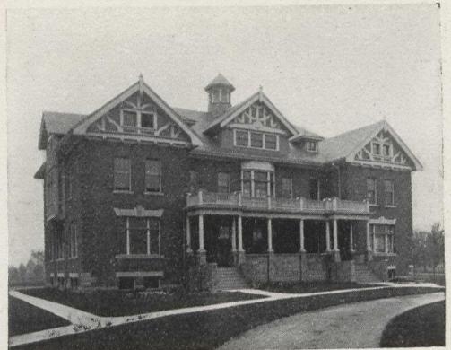
One of the four Cottages, Asylum for Epileptics, Woodstock, Ont. F. Heakes, Architect. Purdy, Mansell Co., Ltd., Plumbers.
