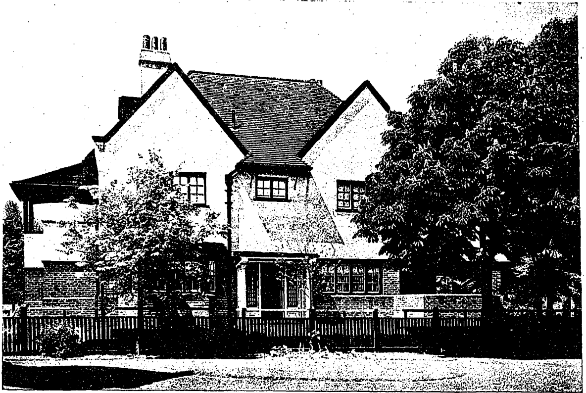
Residence of F. A. Coryell, Jameson Avenue, Toronto. Chadwick and Beckett, Architects.
