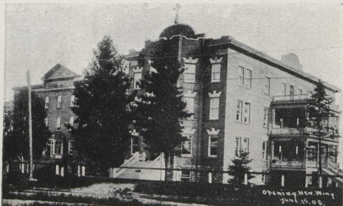
General Hospital, Sault Ste. Marie, Ont. H. W. Angus, Architect. Moore & Brown, Plumbers.
