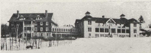
Cottages, Muskoka Sanitarium, Gravenhurst, Ont. Burke & Horwood, Architects. Purdy, Mansell Co., Ltd., Plumbers.
