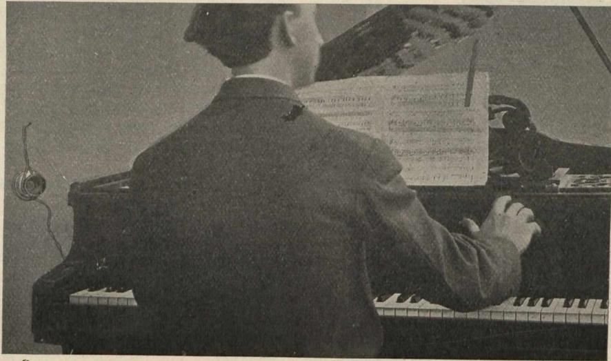
Fig. 2.—Simple Arrangement of Transmitter Suspended on Wall for Transmitting Piano Music.
