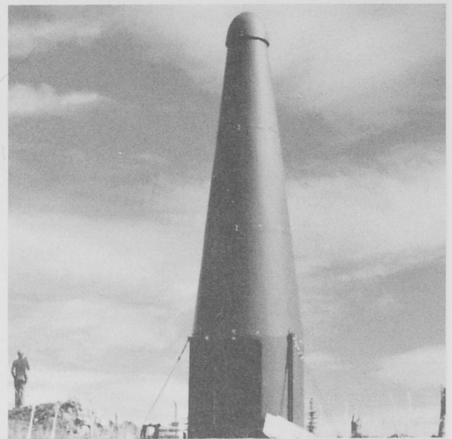
Comshell (communications shelter) covering radio repeating equipment in an area of violent weather, such as on top of a mountain near Cranbrook, British Columbia. Radio equipment and work area are in the lower section, complete with potash battery power source (usually with photoelectric cells that generate electricity from the sun). The antenna is in the upper section.
