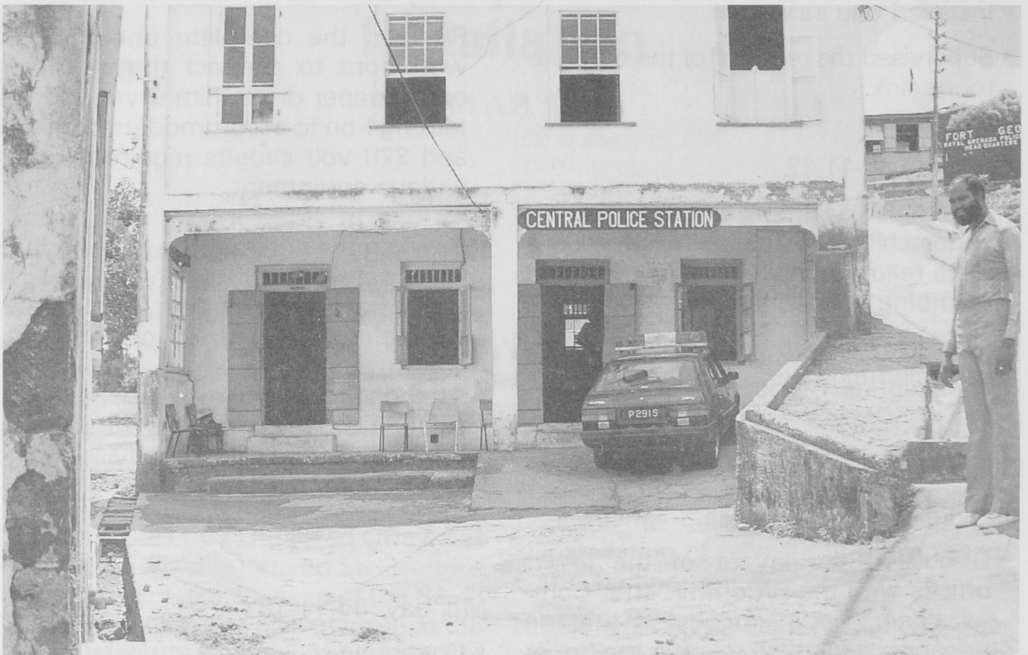
The Central Police Station at Fort George, RGPF headquarters, St. George's, Grenada.
