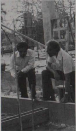
CFTC structural engineer working in Barbados
