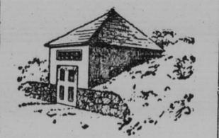
wall for the earth of the bank. The back and sides are laid up in stone to the top of the ground. The rest of the building is wood. A wide door permits a team to be driven, or rather backed, into the building to unload or to load. When laying up the wall at the sides and rear it will be well to lay a line of drain tile outside the stones, to lead away any water that may soak down from the hill above. Half lime and half cement, with sharp sand, makes a good mortar for such stone work.
