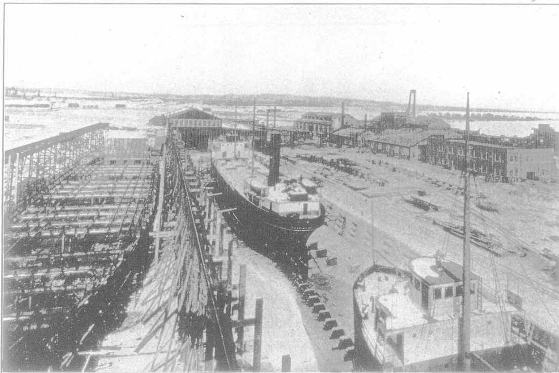
View of Western Dry Dock and Shipbuilding Plant at Port Arthur, showing ships under construction
