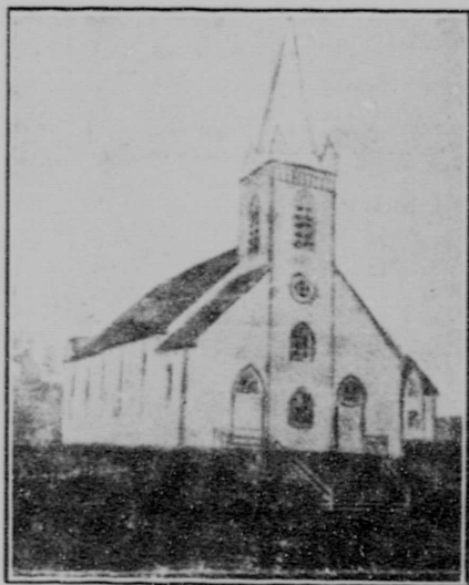
Greenspond Methodist Church.
