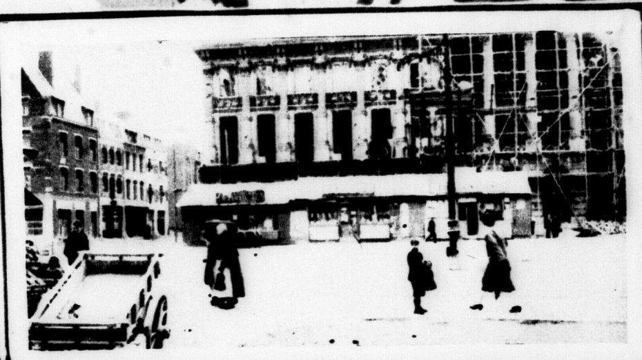
The war-damaged Hotel de Ville (city hall), Cambrai, France, is at last being restored
