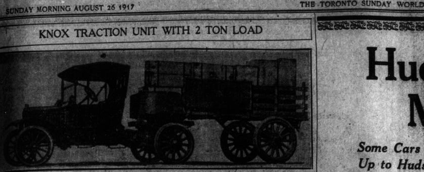
ction Unit is one that makes an especial appeal to the engineer, in that it converts a pleas tractor with semi-trailer, and in so doing imposes no load on the chassis of the car or its was not designed to carry, and at the same time takes advantage of the latent draw bar pull tachment provides the largest hauling capacity for the smallest outlay. The Knox Unit is d vides the largest hauling capacity fo
