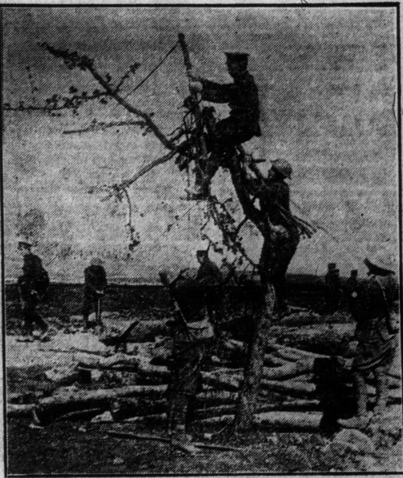
EMERGENCY TELEPHONE POST. The Canadian Engineers across the waters sometimes have to use just an old wreck of a tree for their telephone posts, as in the case of the emergency post seen in the picture.
