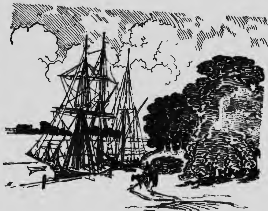
THE HARBOUR, GATEHOUSE
