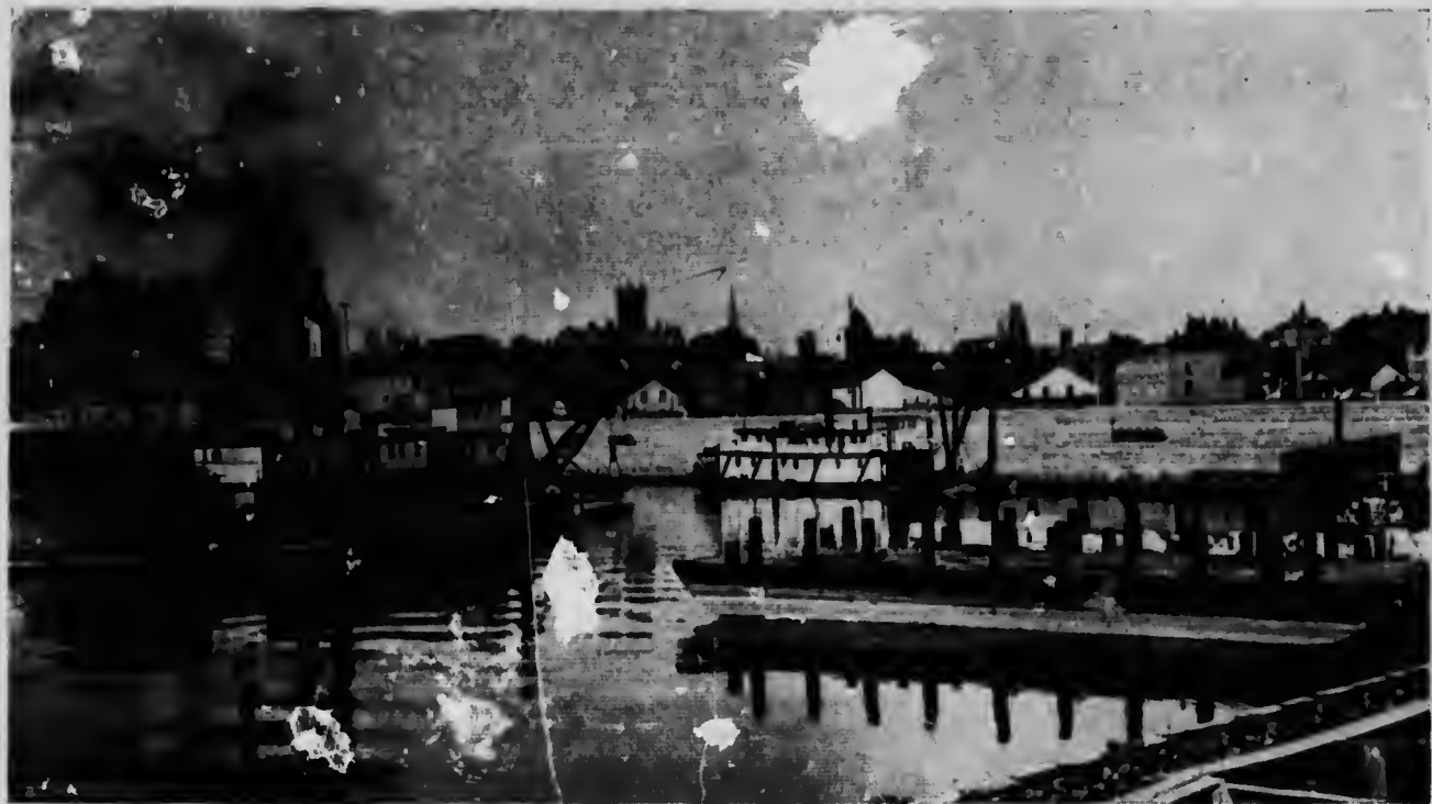
The Retaining Wall for Causeway across James Bay, Dredge King Edward VII. in foreground.
