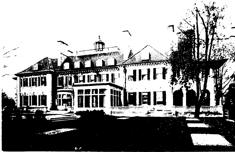
RESIDENCE OF SIR JOHN C. EATON. Wickson & Gregg, Architects.
