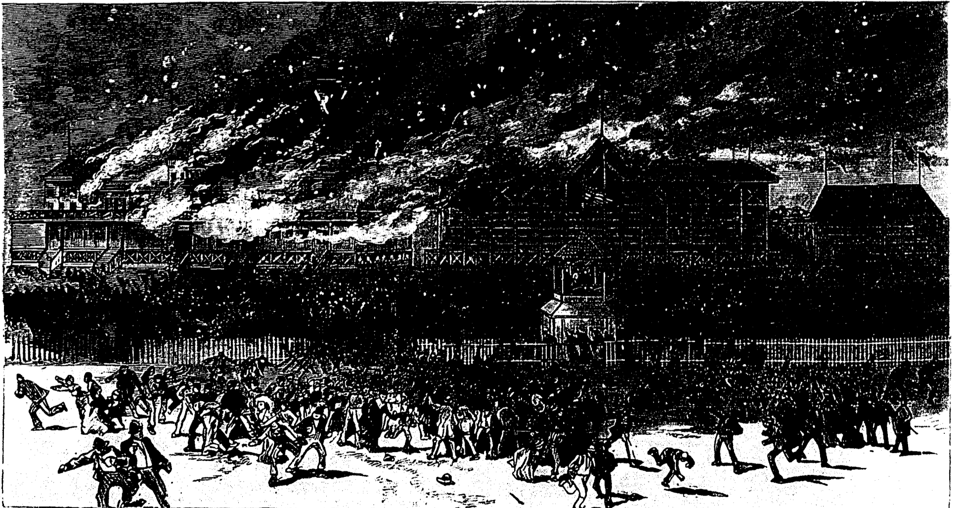
THE GRAND STAND AT THE EXHIBITION GROUNDS, KANSAS CITY, DESTROYED BY FIRE, SEPTEMBER 14TH.
