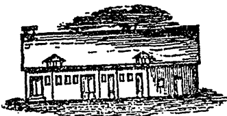
No. 5.—View of the Shops.
