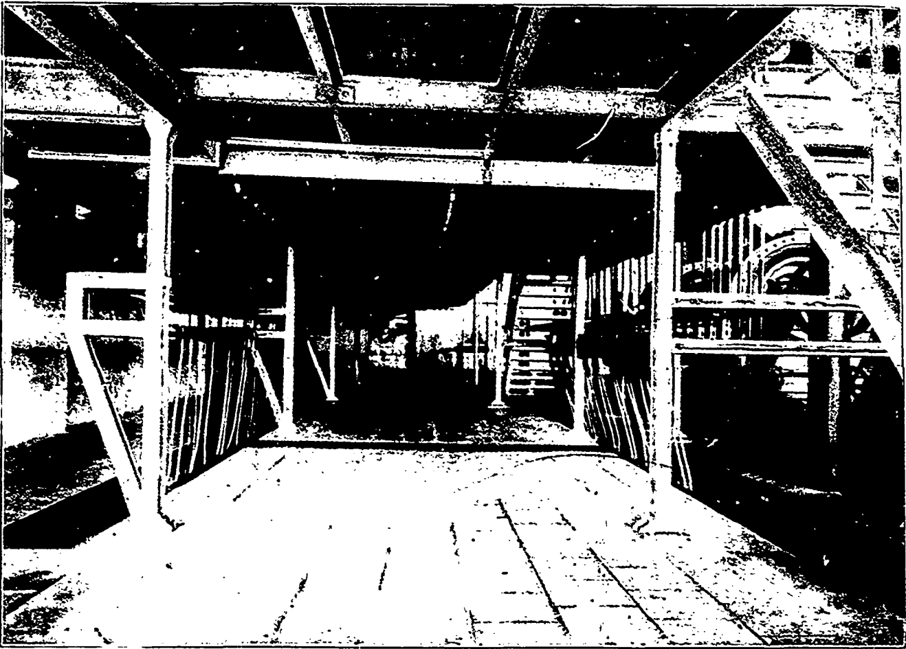
SPACE UNDERNEATH SWITCH-BOARD, SHOWING WIRES FROM GENERATORS, ROYAL ELECTRIC COMPANY'S ALTERNATING LIGHTING STATION, MONTREAL.
