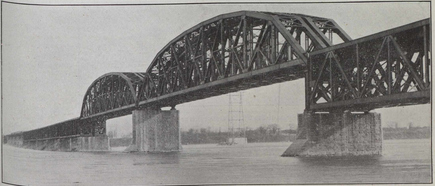
The Channel Spans of the St. Lawrence River Bridge.
