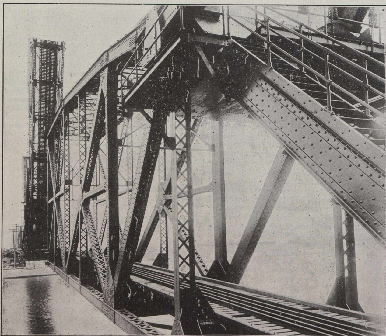
The C.P.R. Bascule Bridge at Sault Ste. Marie with One River Arm Fully Opened.
