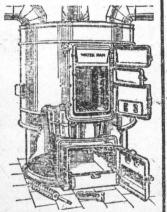
The walls of the fire-pot are straight and ashes do not bank against them to stop the radistion of heat from the burning coal. The doors of
