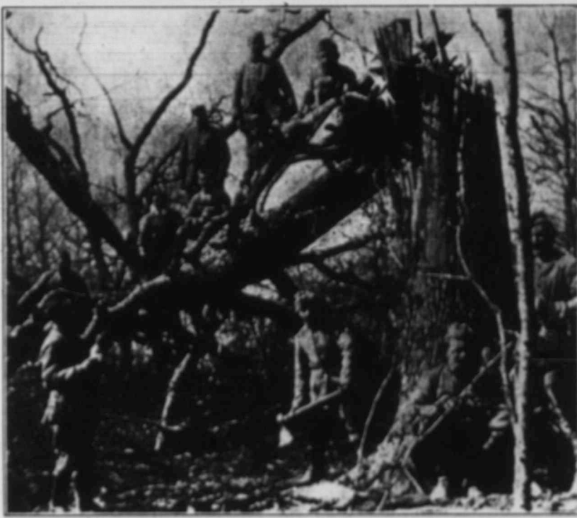
The Yarkas region is covered with stumps and broken trees that were cut down by shell fire. Here is a wood near Vancouver.
