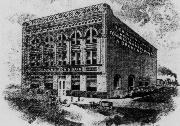
BANNATYNE ST. EAST TRANSFER TRACK.
