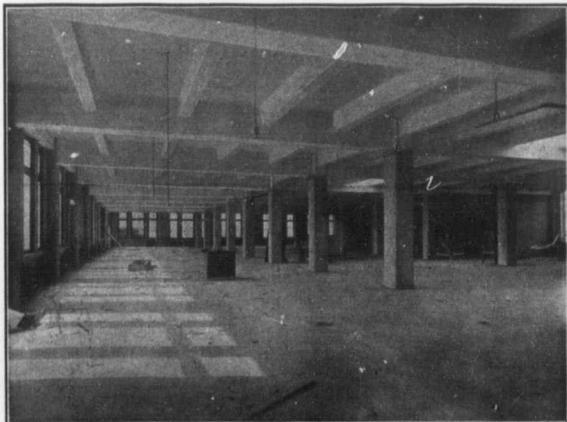
A section of one of the manufacturing floors of the new Book Room—note the size, the steel and concrete construction and the splendid lighting. This room, which will house the Bindery, is 100 feet wide by almost 200 feet long.
