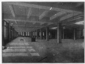
A section of one of the manufacturing floors of the new Book Room steel and concrete construction and the splendid lighting. This room, which will house the Bindery, is 100 feet wide by almost 200 feet long.
