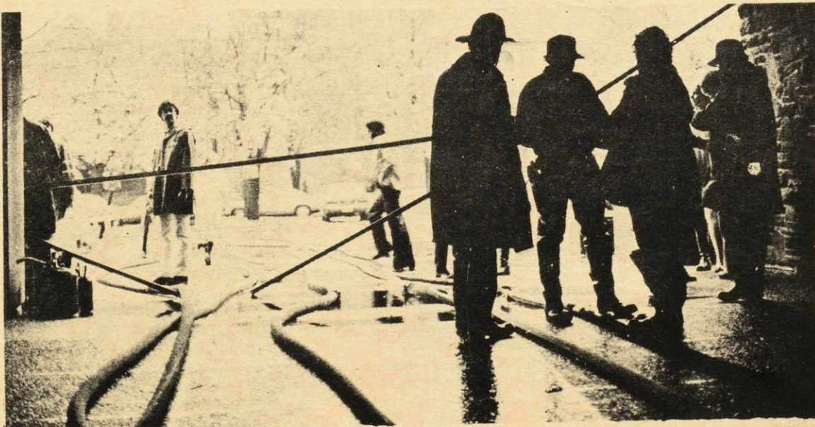
A broken water main caused severe flooding in the basement of the Killam Library which in turn left the Chemistry building and Howe Hall without lights on Friday and early Saturday morning. Library staff report that no extensive or serious damage resulted although it took time for the machinery to dry out.
