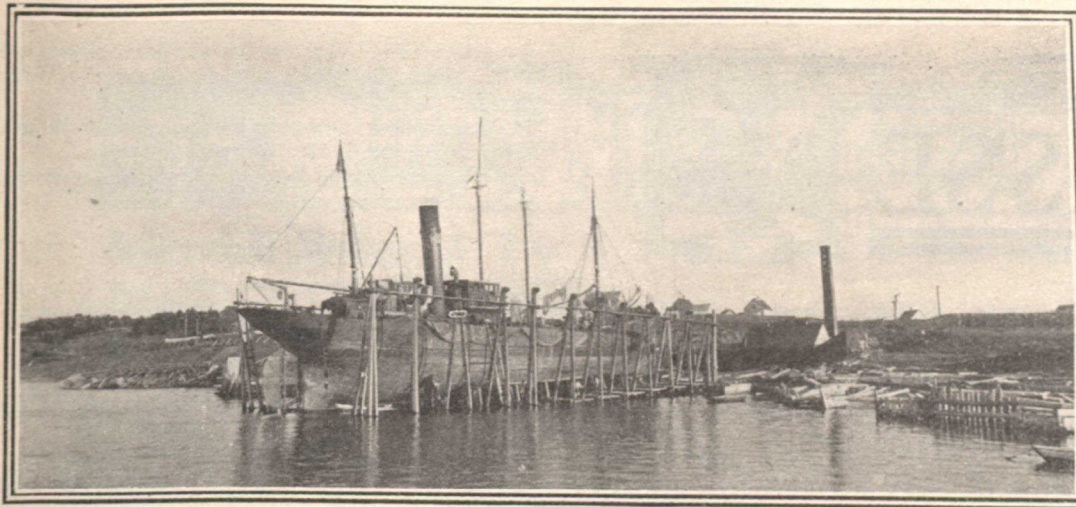
Steamer at the Marine Yards at Point Tupper, N.S., hauled up ready for repairs
