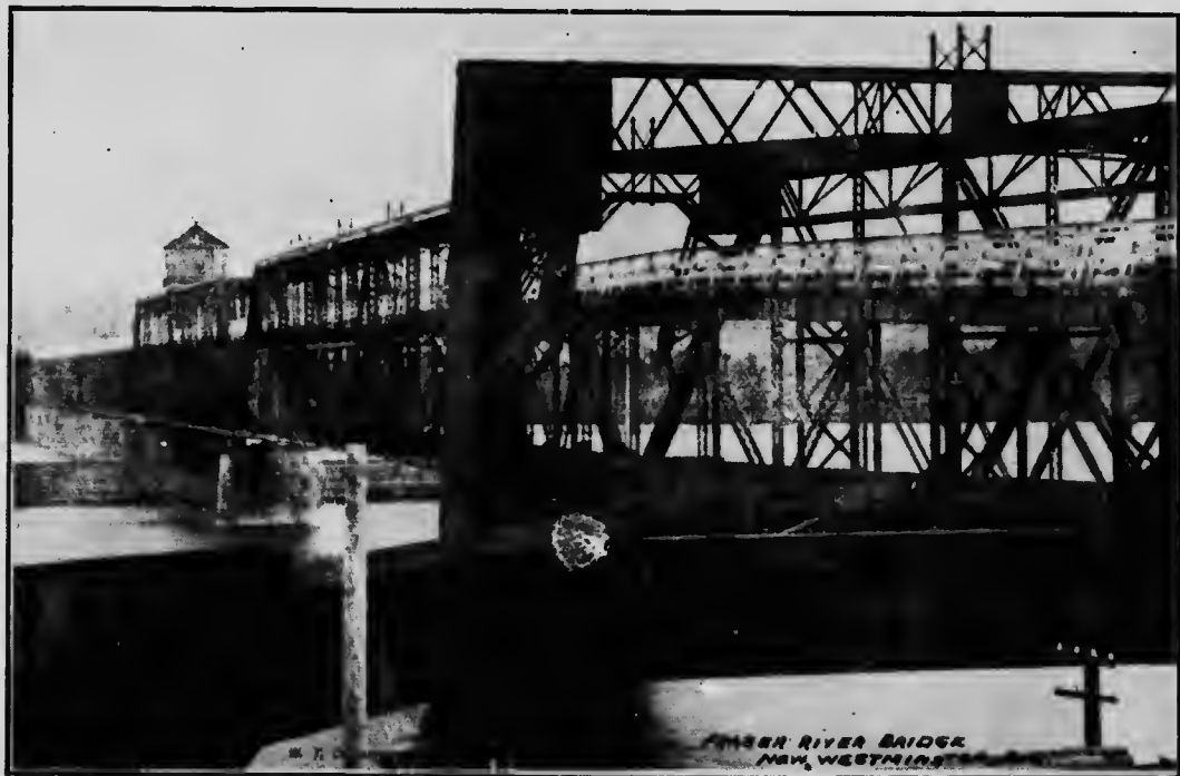
Fraser River Railway and Traffic Bridge—1781 feet from shore to shore; width, 19 feet; length of draw, 350 feet; traffic roadway, 26 feet above railway; cost, $1,000,000. This gives admission from the south to one of the great transcontinental lines—the Great Northern Railway; and it is expected that at an early date the Northern Pacific and other railways from the south will make use of the same highway to reach the business end of B. C.
