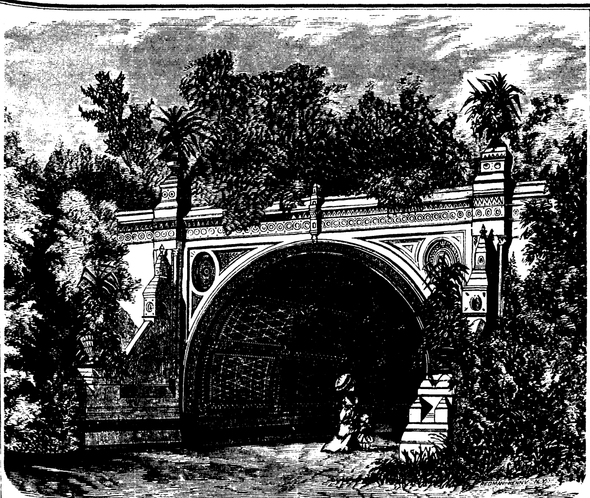
CLEFTRIDGE SPAN, ERECTED OF BETON COIGNET, IN PROSPECT PARK, BROOKLYN, N. Y.
