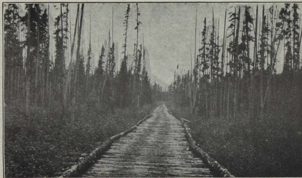
A stretch of Corduroy west of Halfway on the road to Wasapika.
