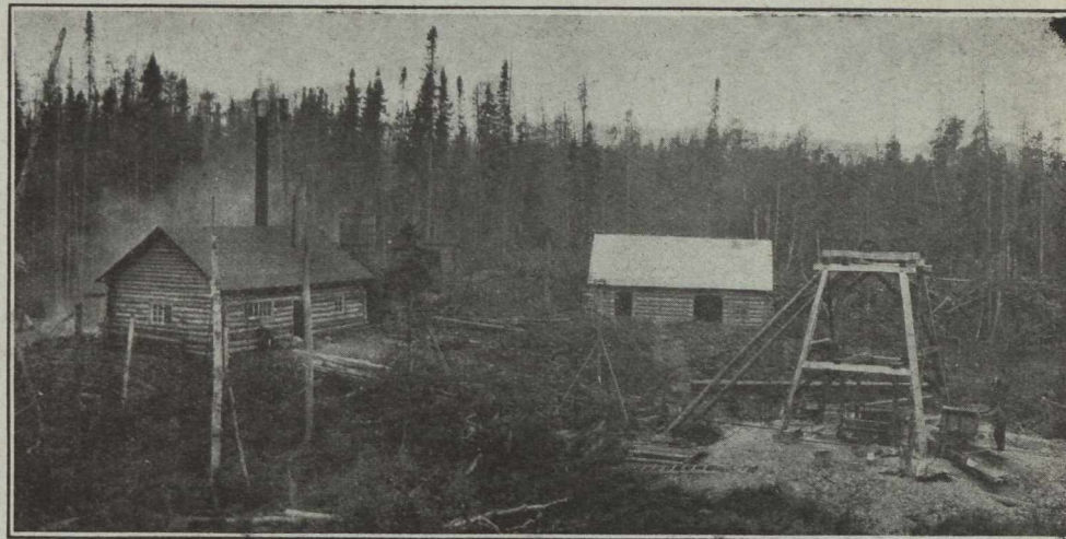
The Wasapika Power House and Head Frame.
