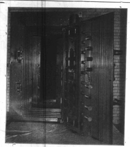
Vault doors in Bank of Montreal and Royal Trust Company, Montreal Three times larger and heavier than any other in Canada. Doors and Vestibules weigh 60 tons. Total weight of lining and doors 260 tons. Accepted to be the finest piece of vault work in construction and workmanship in the Dominion. — Built by the old established firm of
