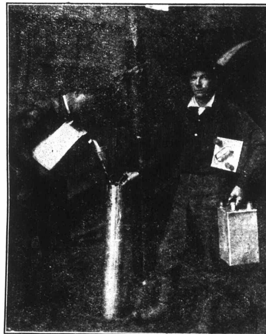
POURING THE NITRO-GLYCERINE IN THE HOLE PREPARATORY TO SHOOTING AN OIL WELL.
